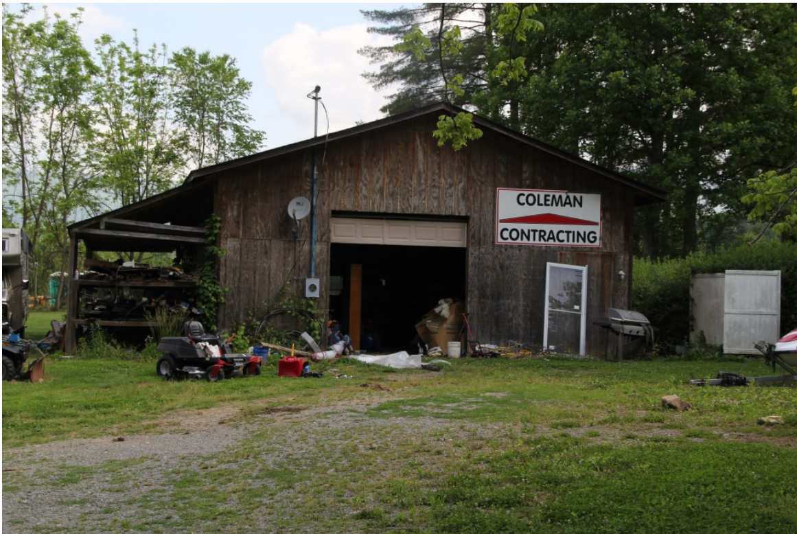
Workshop, façade, view to north
