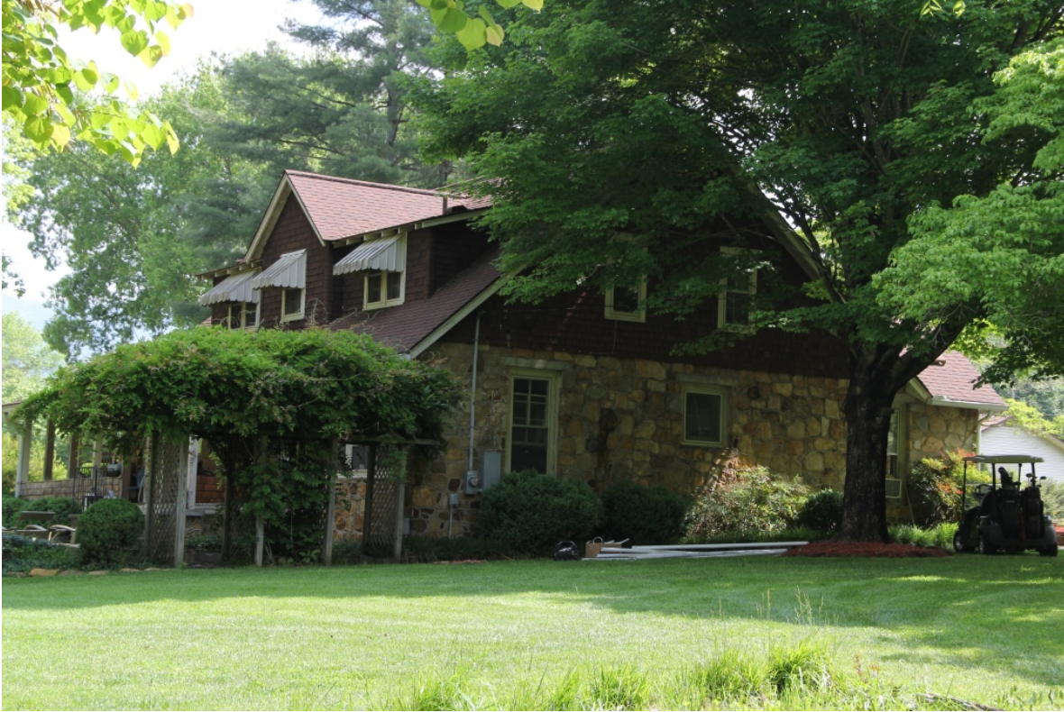
Bristol House, oblique rear view to northeast
