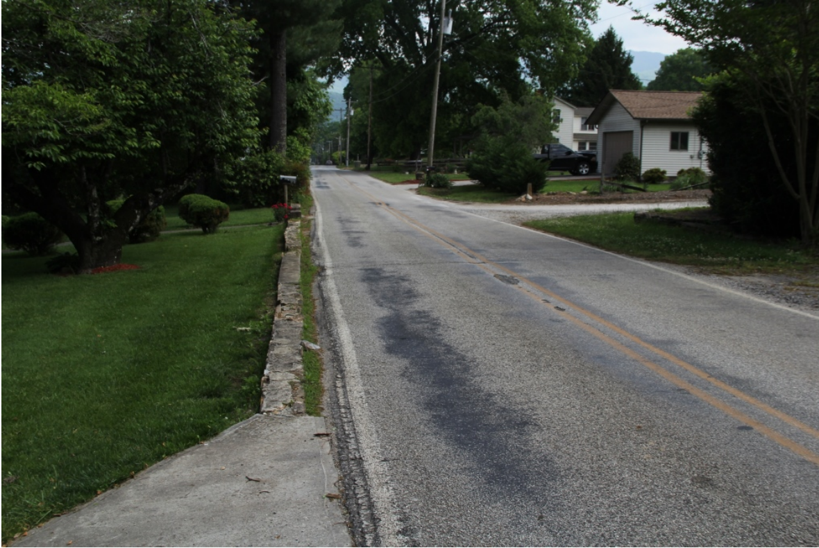
Stone border wall, view north along Bristol Avenue
