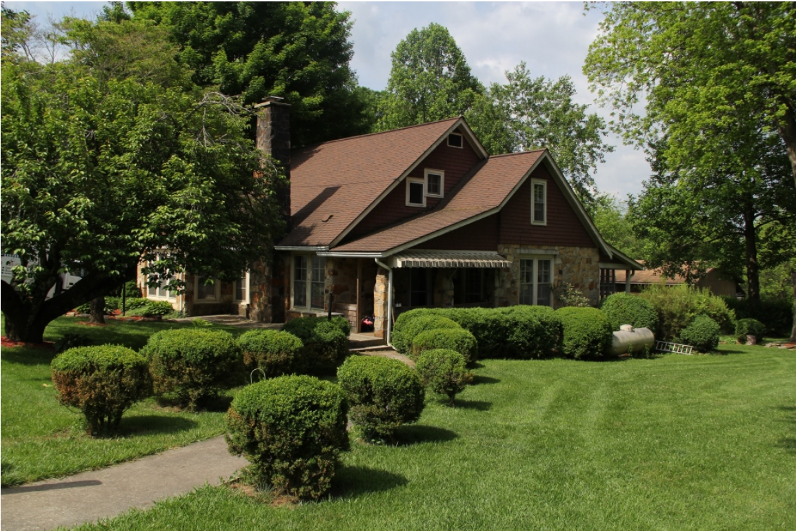
Bristol House, oblique view to southwest
