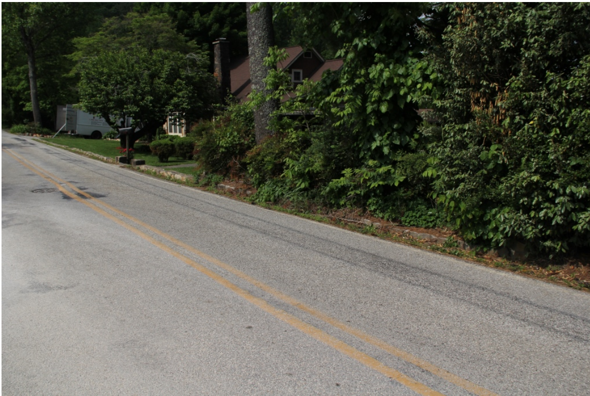
Stone border wall, oblique view to southwest
