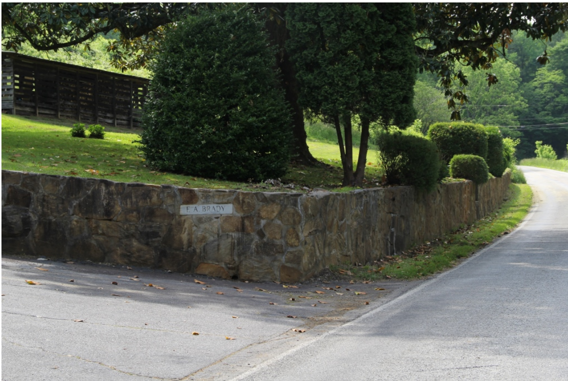
Brady House, 455 Bristol Avenue, stone wall, view to southeast
